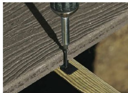
Hidden Fastener Installation to Joist
