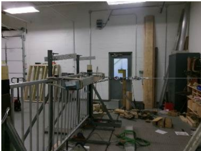
Photo No. 3 Horizontal Uniform Load Test on Top Rail
