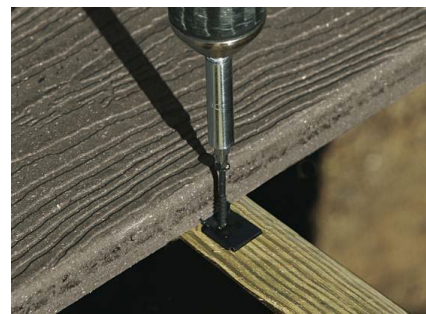
Hidden Fastener Installation to Joist
